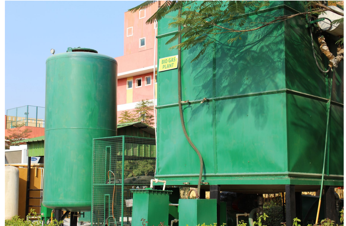
Bio-Gas generation system 30kg of Gas per day with 500 kg of Kitchen waste
